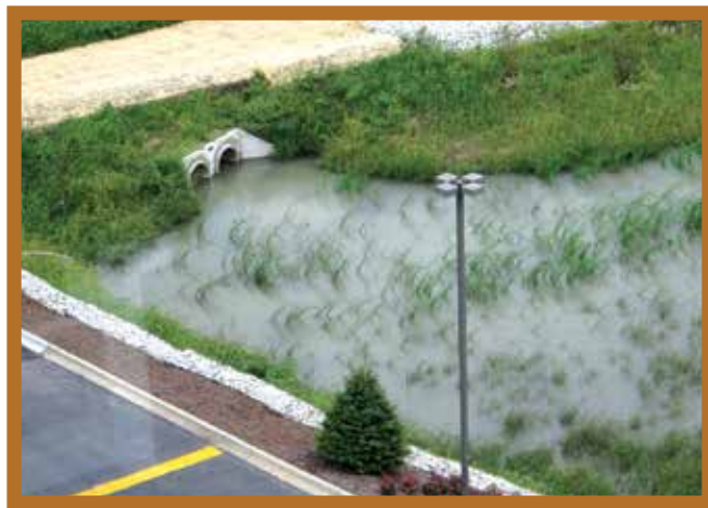
When Walmart built in the Pullman area, consistent with their emerging green building practices and with local ordinances, they created stormwater capture capacity on site.
