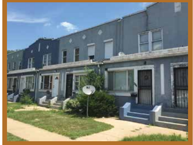
Top: George Pullman was both the developer and the landlord in Pullman, providing sturdily-built rowhouses such as these. When U.S. Steel founded Gary, Indiana, in 1906, the company tried to stay out of the real estate development and rental businesses, having learned that Pullman-style paternalism can breed resentment on the part of employees. Bottom: The "Edison Concept" Polk Street Terrace homes were built and initially managed as rentals by the Gary Land Company, a subsidiary of U.S. Steel, to provide quality affordable housing to incoming skilled workers from other U.S. Steel facilities.
