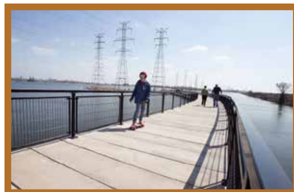
Exciting new regional trails like the Wolf Lake Trail connect natural areas with industrial landscapes.
